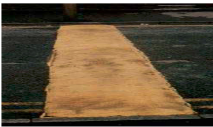
Yellow Thermoplastic 'Thump' Cost per feature = £500 (approx) -----
