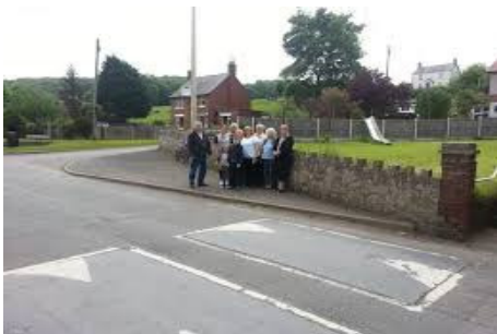
Speed Cushions Cost per feature = £500 per pair (approx)
