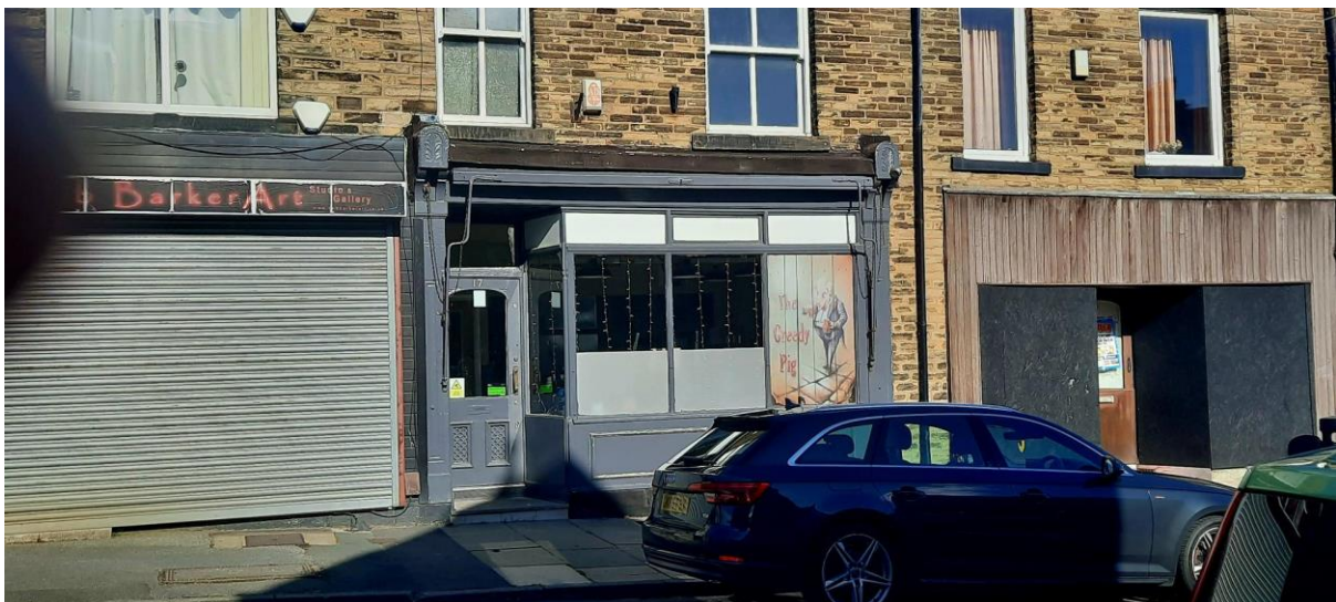
Example of a traditional shopfront alongside less sympathetic modern replacements on Stony Lane
