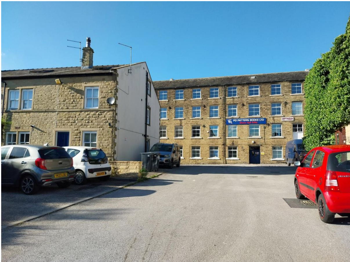
Whiteley's Mill (also known as Stone Hall Shed/Mills) was a worsted mill. It is still in commercial use. The cottages in front of the mill were most likely built for textile workers.
