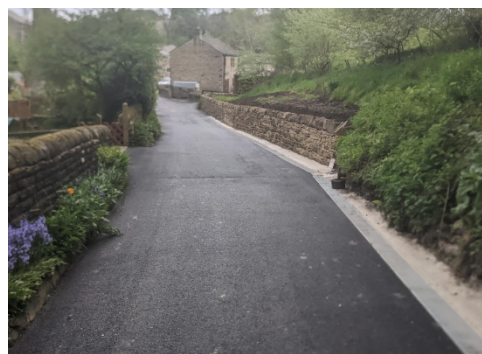
Lund Lane Resurfaced with flood channel installed
