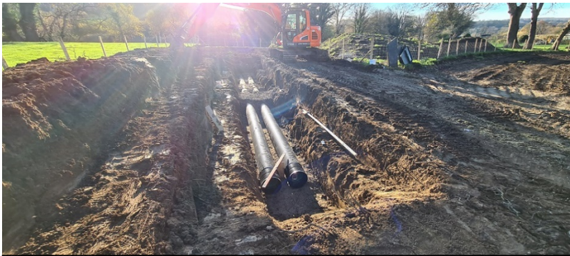
Installation of flood relief pipework
