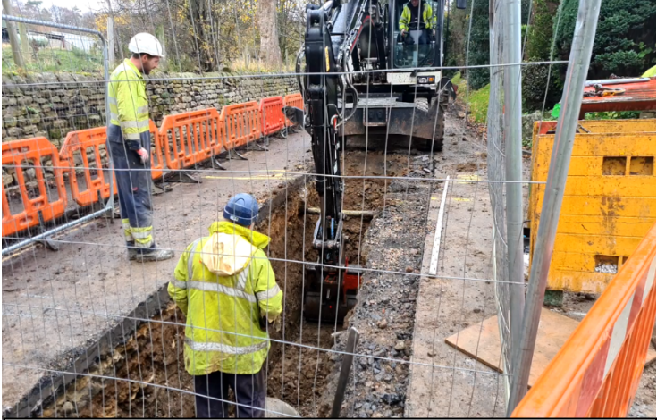
Restricted working room casued logistical challenges
