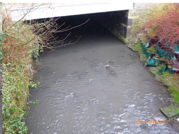
At Ambler Mill, near Forster Retail Park, 17 th Feb
